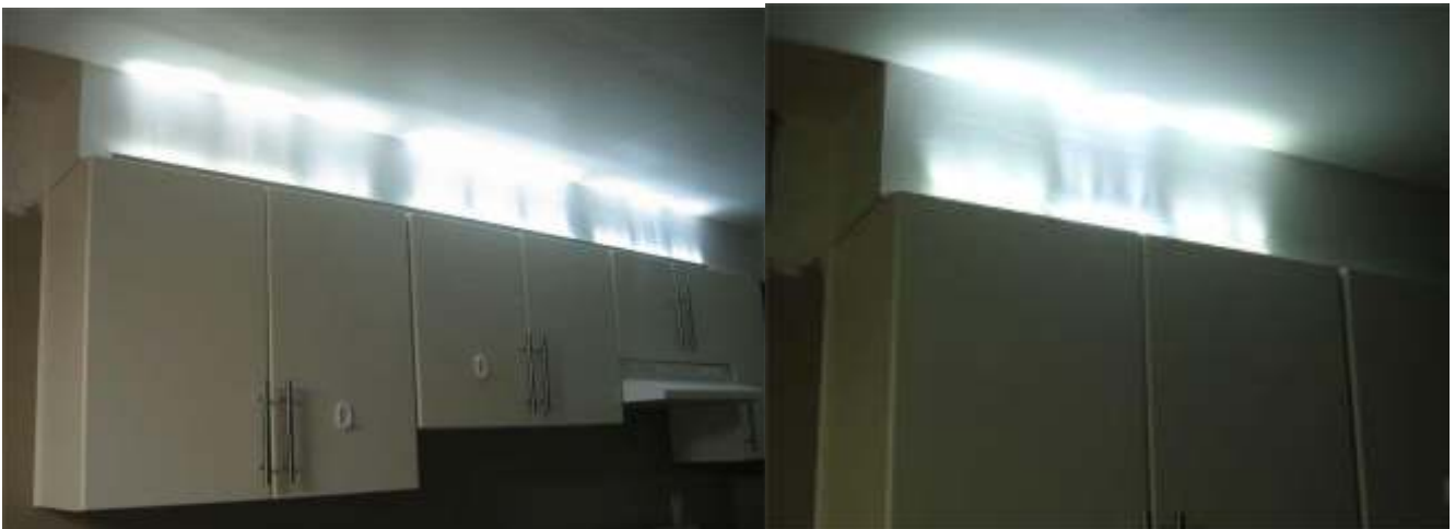
LED light strip for lighting.
