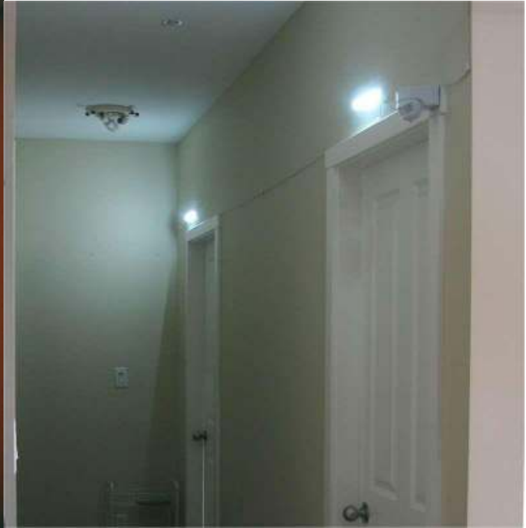
Corridor lighting with PIR motion sensor.
